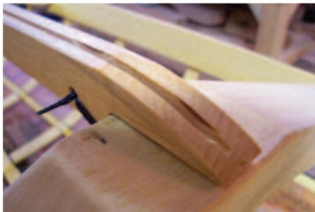
*The cockpit ends of the stringers feather out to nothing. The groove should be brought flush to the bottom of the stringer (perhaps cut  $\frac{1}{8}$ " into the deck beam?)*
